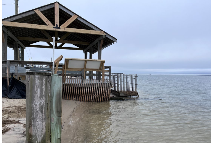
Pavilion and boat ramp
