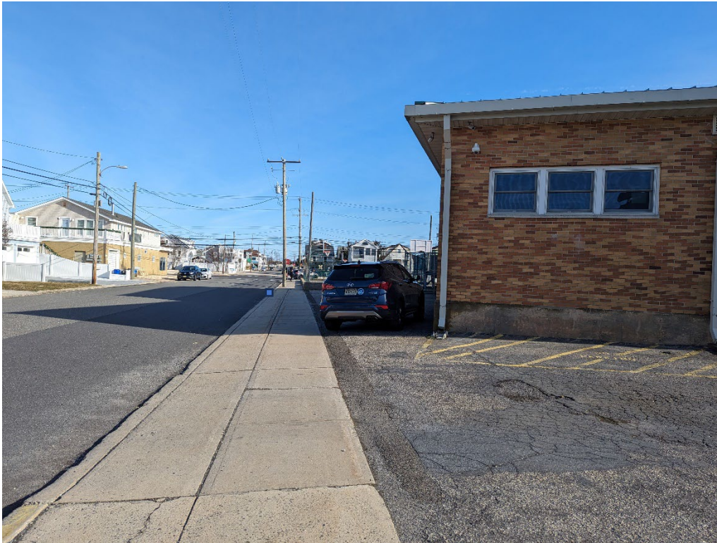
Image 4 - View toward Central Avenue, overflow vehicle parking
