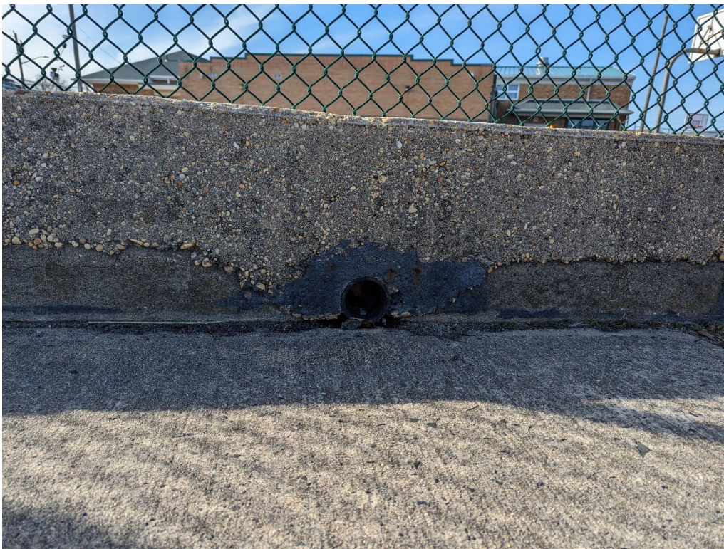
Image 7 - Drainage pipe from the Study Area to the sidewalk
